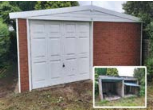
Hanson Garage Refurbs Pages 28-29
